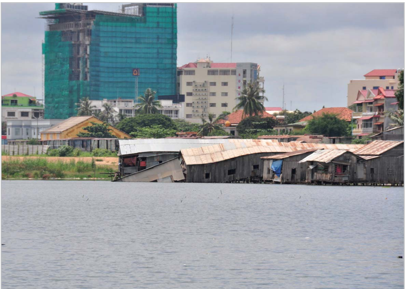
Houses collapse into Boeung Kak lake after sand is pumped to reclaim land for commercial development
