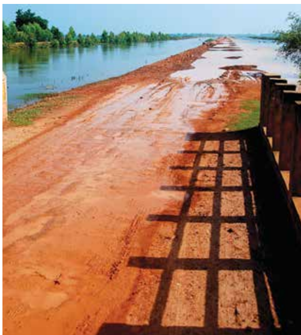
Flooded road to Trapaing Thma dam, Pnom Srok district, Banteay MeanChey (Photo - Humanitarian Response Forum 2013)
