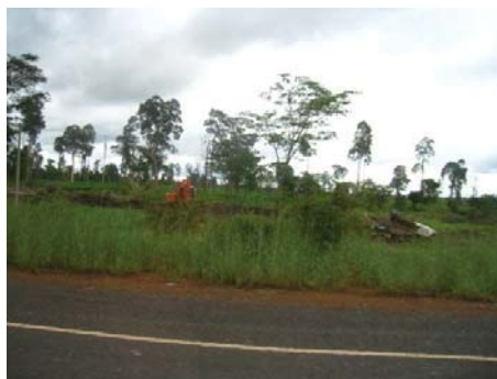
Land clearing activities
