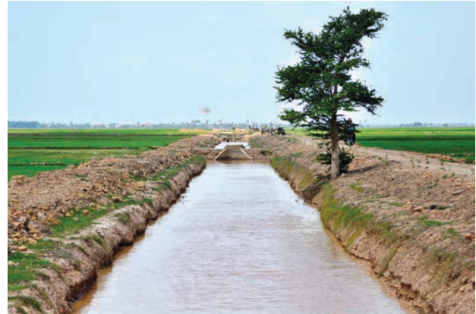
Sweden-funded canal restoration allows farmers in Chong Ampil commune, Prey Veng province, to increase rice farming, improving their resilience to climate change impacts. Photo: UNDP Cambodia
