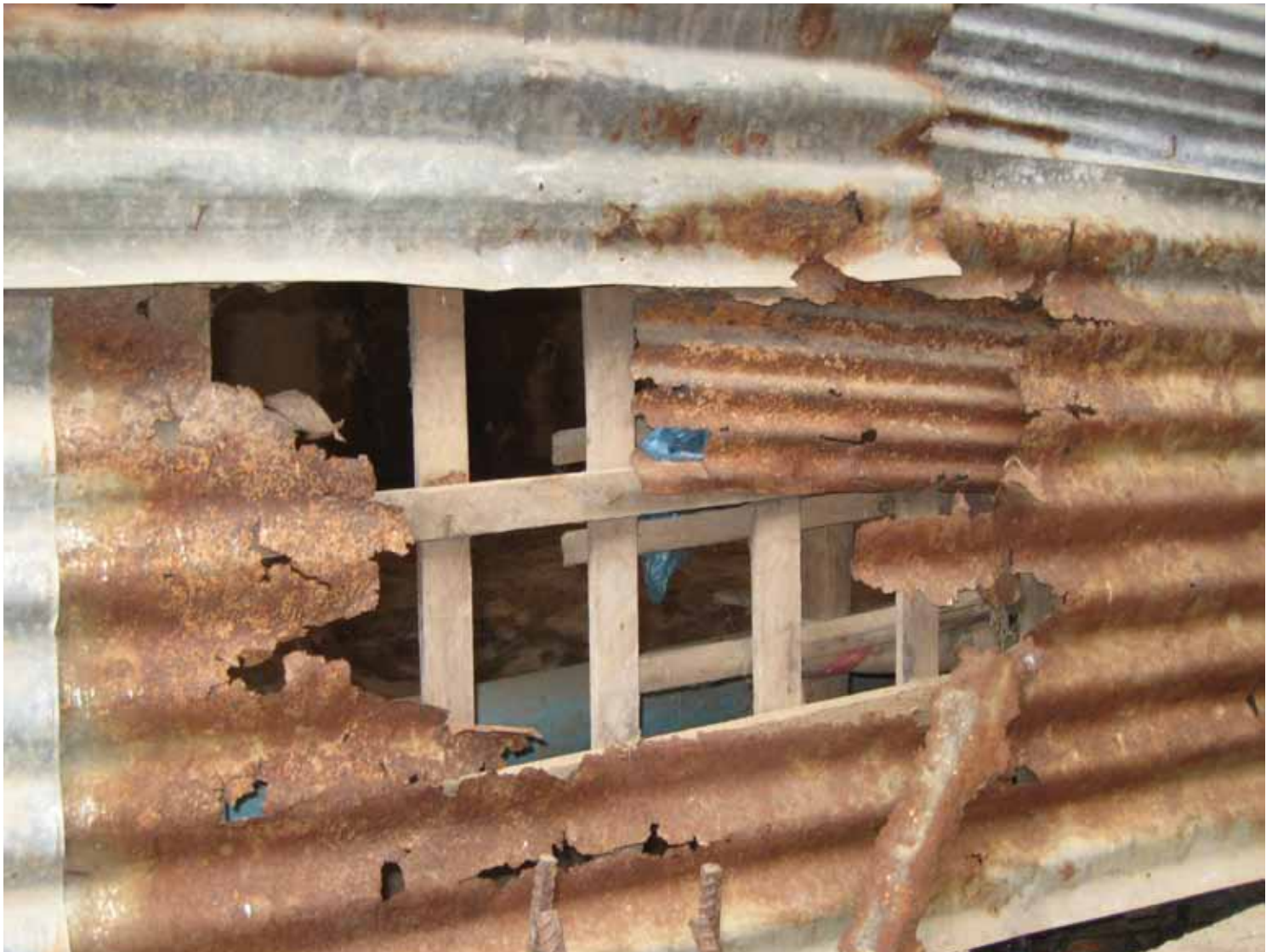
05 - hole in house wall
