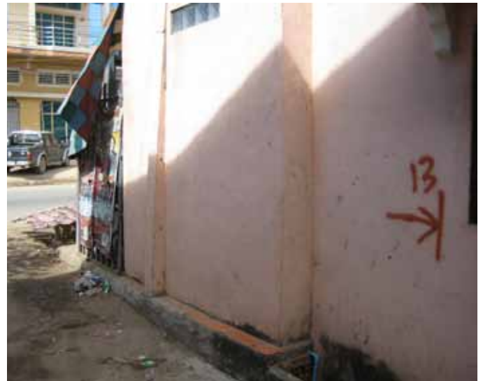
13m spray paint markings on house holds
