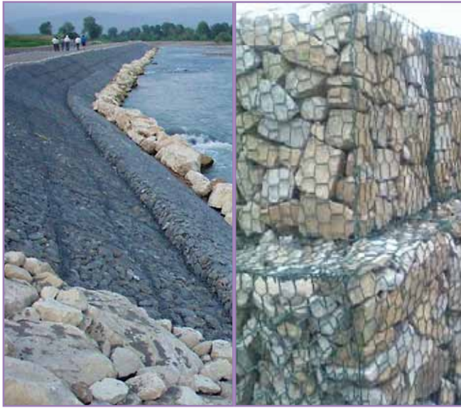
gabion river embankment
