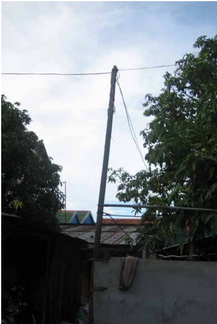
01 - unstable / makeshift electrical poles
