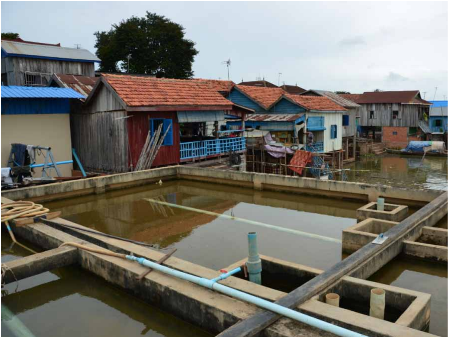
03 - private water plant - khor village
