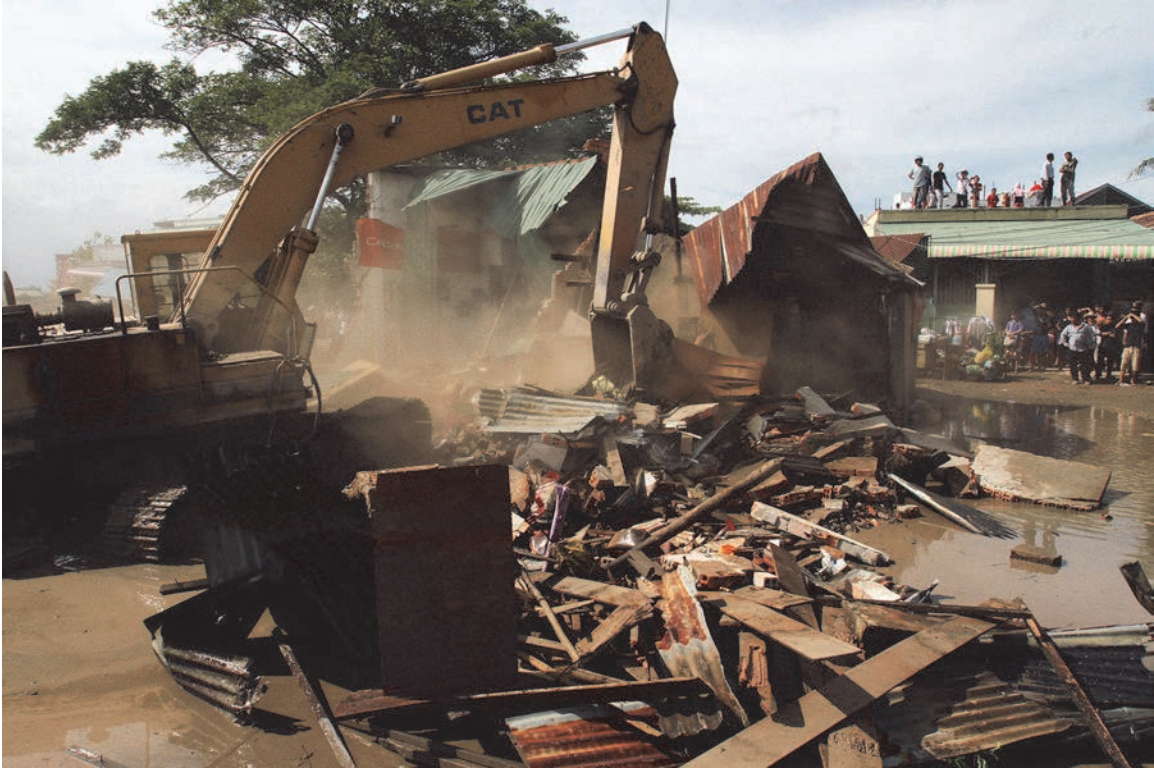
People look on as a house is demolished at Boeung Kak Lake in Phnom Penh on September 16, 2011.
