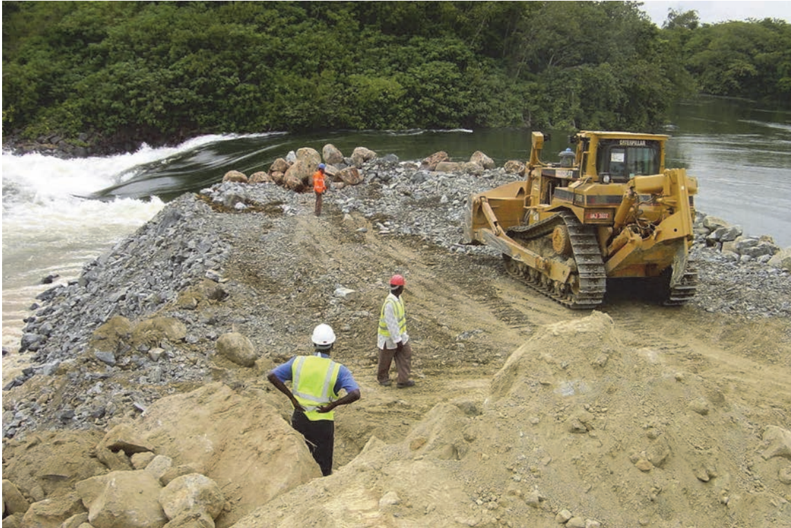
Construction efforts associated with the Bujagali Dam in 2007, a World Bank-funded hydropower project in Uganda. NGOs critical of the project have been subjected to pressure from the Ugandan government to drop the campaign. © 2007, AFP
