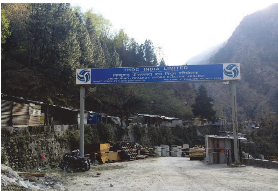
Project site of the Vishnugad Pipalkoti Hydroelectric Project in Uttarakhand, India, a hydropower generation scheme on the Alaknanda River financed by a US$ 648 million loan from the World Bank. © 2014, Human Rights Watch
