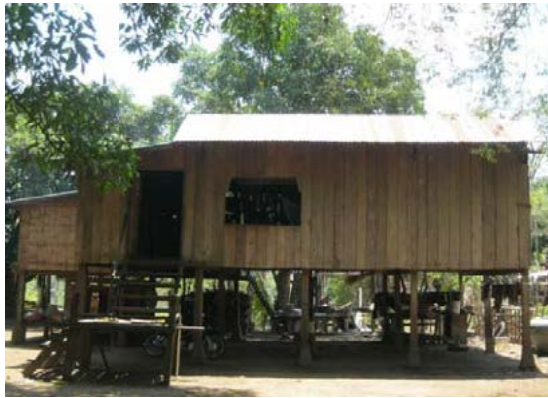
Picture 1 - Wooden house with zinc sheets roof which is popular in the study areas
